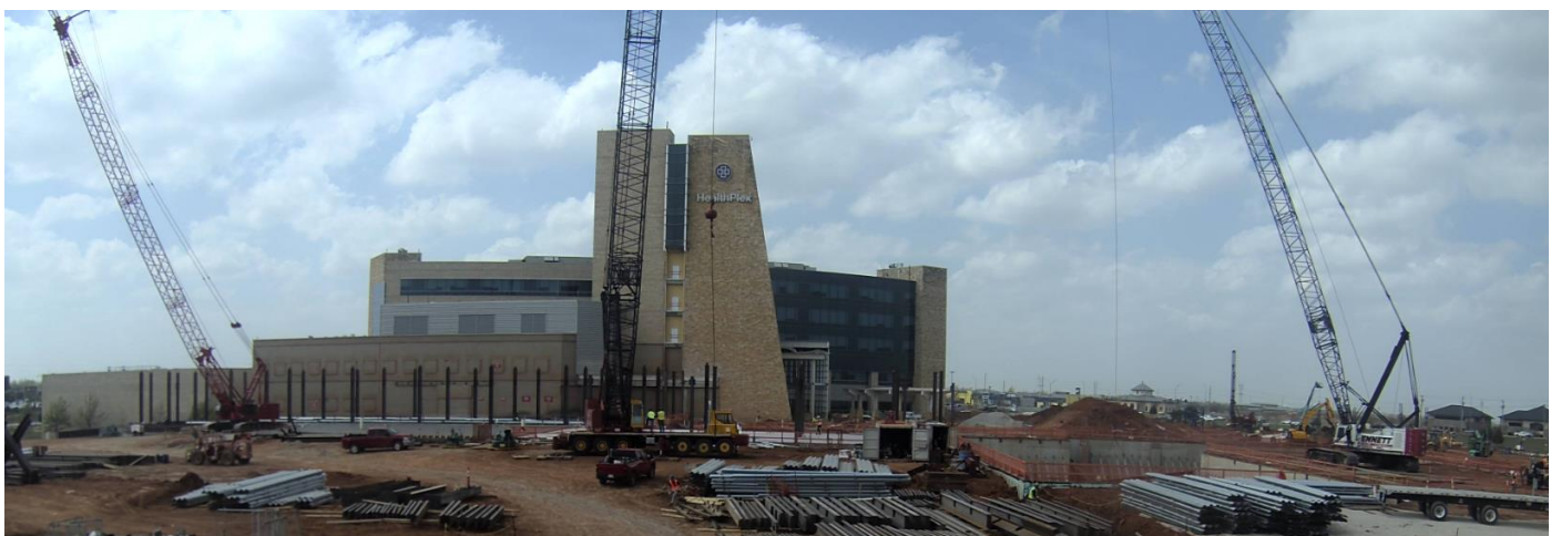
Three Crawler Cranes working on the HealthPlex.
