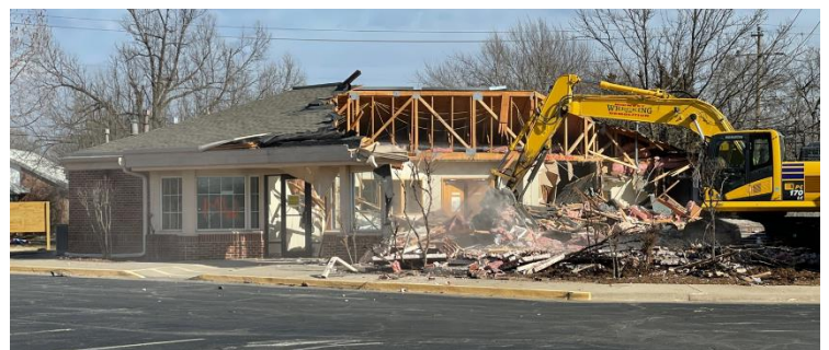
Demolition of Nu-N-Nuf Thrift Shop
