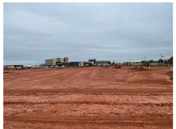
Parking Lot A Construction Underway!
